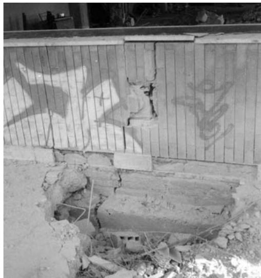
Figure 2. Crack passing on foundation of grade beams, with a horizontal translation of 4 cm.
