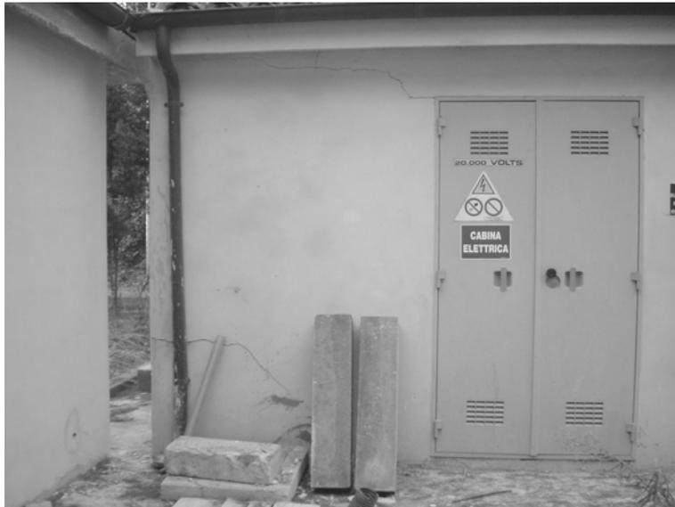
Figure 6. Cracks for a flexion cut-off combined action of a new handwork used as an electric cab, next to the principal building.
